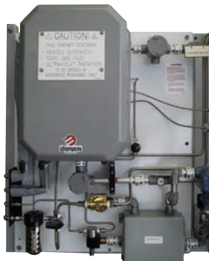
BRM 961-AGX Acid Gas Analyzer System Oven Back Panel - Oven Closed Rev 0
